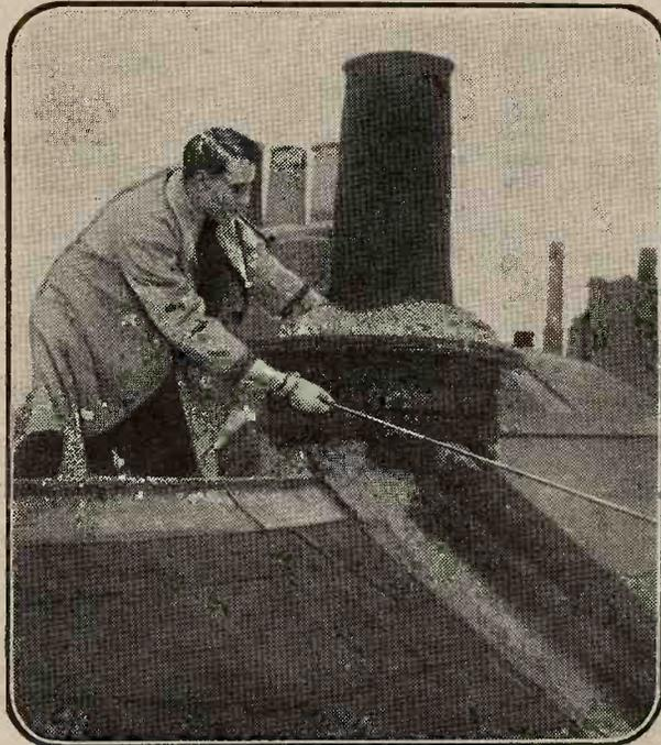
A chimney stack will make a good support for your Aerial. Care should be taken that the rope does not fray against the brickwork.
