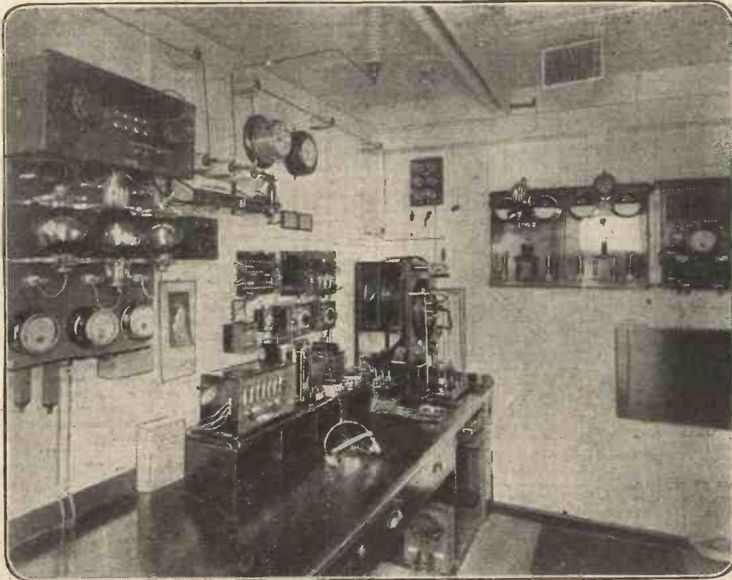
Our photograph shows the wireless installation on the s.s. Arundel Castle. Note the three transmitting valves on the extreme left, and just below them the seven-valve Marconi Amplifier, and the Type 31 Crystal Receiver. On the extreme right is the "spark" transmitter. A quenched gap is used. The "change over" switch for connecting one or another transmitter to the aerial is seen a little to the left of the first clock.
