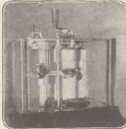
The Vibrometer, for measuring vibration frequencies.
