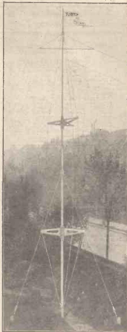
Photo of the Patent Turret Oregon Pine Cantilever Mast designed by Naval Experts.
