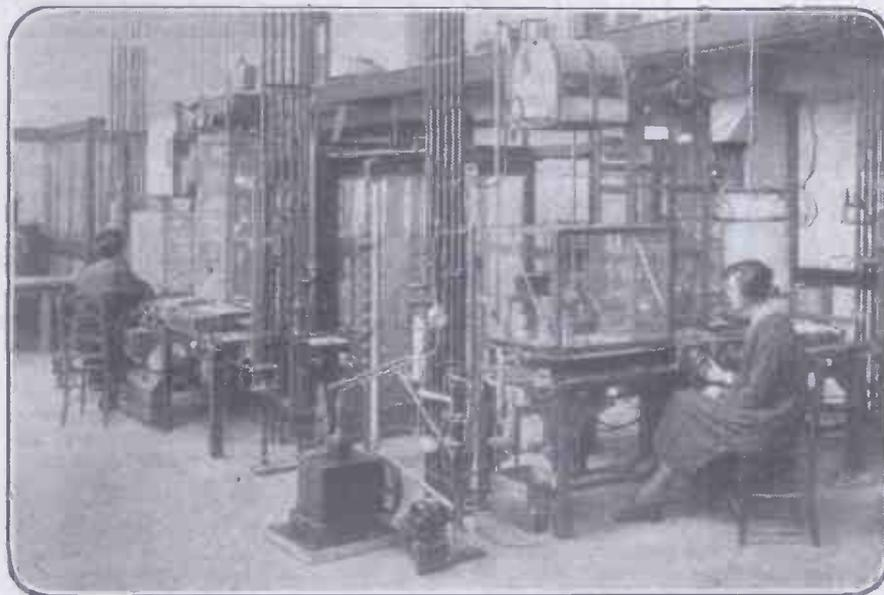
Testing Valves in the G.E.C. Laboratories, Wembley. The valve under test has a pressure of 5,000 volts D.C. on the plate.
