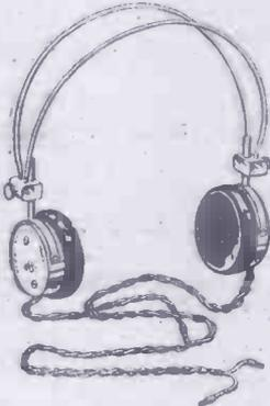
Fitted with Patent Duplicating tags and patent head-bands, and sliding adjustments, most comfortable to wear. Parts are silver and nickel plated. Marked B.B.G.
