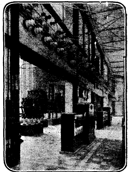
A section of the engine hall.
