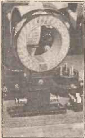
In order that there shall be as little inter-linking as possible between the two circuits, the coils should be aligned as shown in the accompanying photograph.
