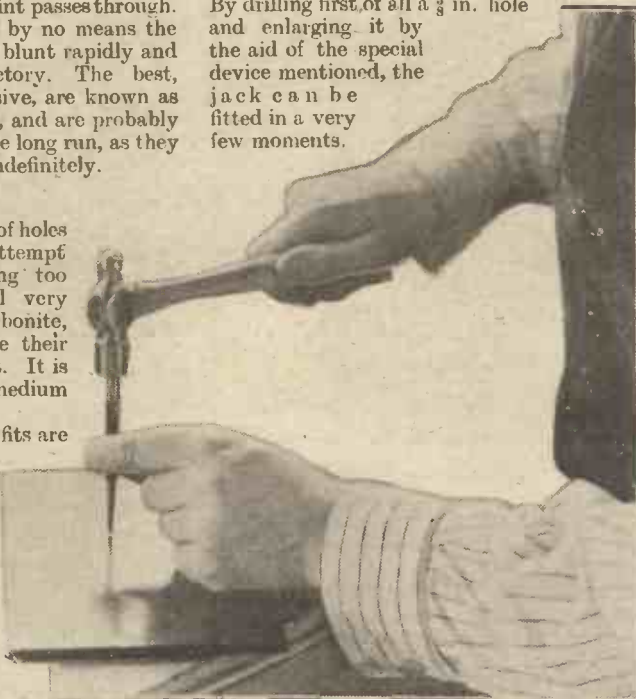
Always use a centre-punch to give a depression for the point of the drill. This saves drill wandering and inaccuracy.
