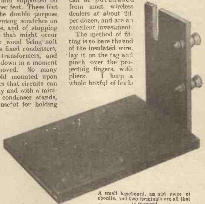
A small baseboard, an odd piece of ebonite, and two terminals are all that is required.
