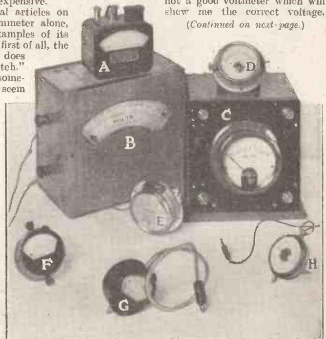
Some of the meters in my laboratory. A.—A "Universal" meter, measuring milliamperes, amperes and volts. B.—A high resistance voltmeter for measuring H.T. voltages. C.—An A.C. voltmeter. D.—A D.C. ammeter (low reading). E.—Hot wire ammeter for transmission experiments. F, G, and H. Portable voltmeters and milliammeters.
