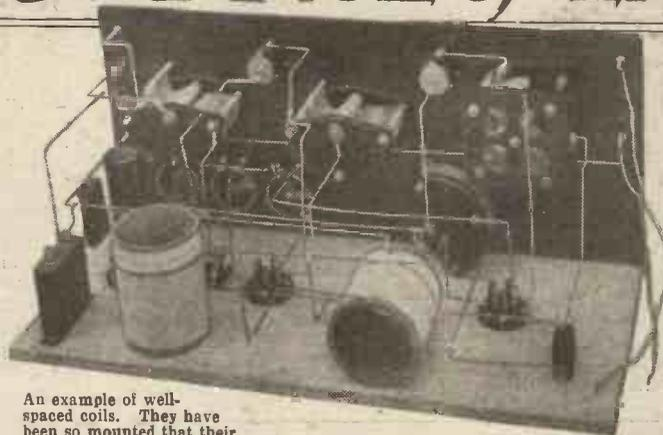
An example of well-spaced coils. They have been so mounted that their magnetic fields will not interact.
