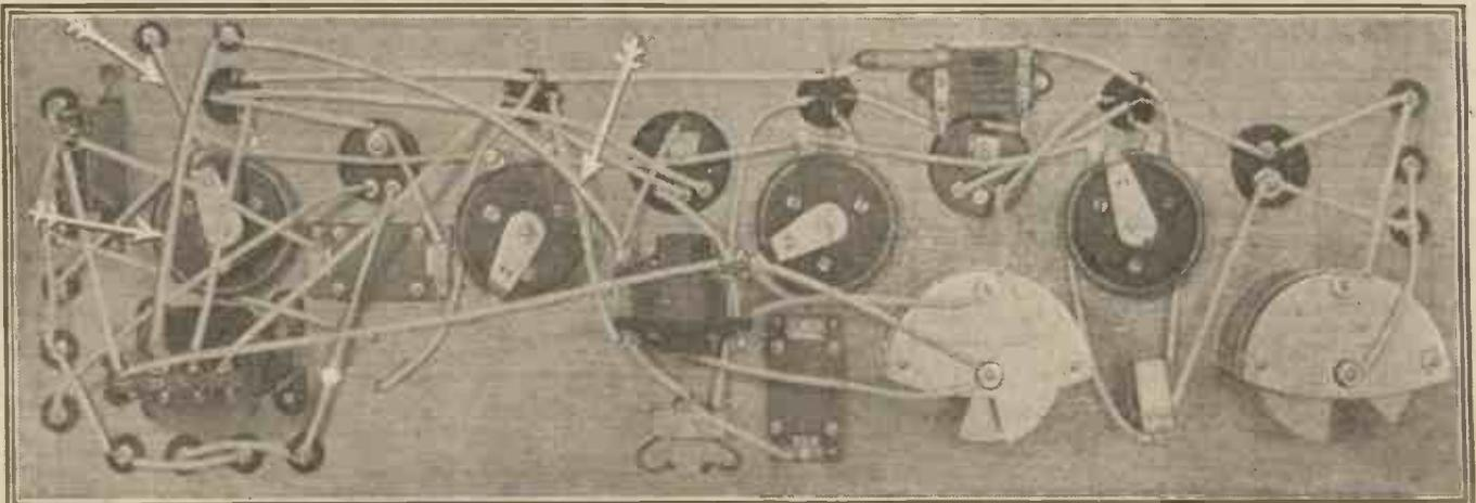
A photograph of the original set, with arrows showing the changes necessary for applying grid bias to the note magnifying valves. Note the two additional terminals marked "G.B." in the heading photograph.
