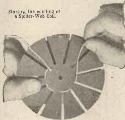
All that is necessary is to make one or two holes in the former and thread the beginning of the wire through these, to make it fast.
