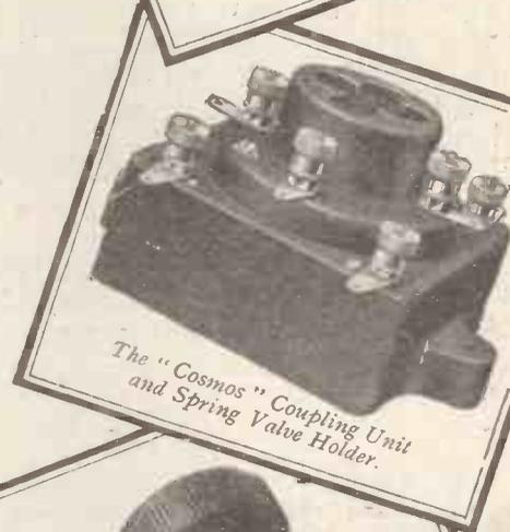
The "Cosmos" Coupling Unit and Spring Valve Holder.
