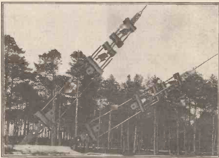
The special mooring arrangements of the bracing cables for the lattice masts.
