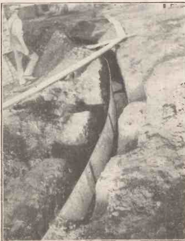
A section of the elaborate earthing system being installed at the new Air Ministry radio station at Mitcham.
