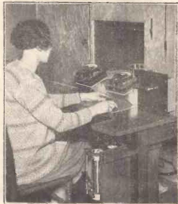
A photometer for measuring the performance of electric lamps and radio valves in which a photo-electric cell takes the place of the human element.
