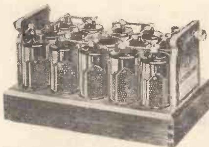
The Hart Rado, a 30-volt H.T. accumulator unit, with the capacity of 3 ampere hours.
