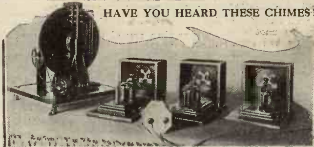
In between items the Bratislava broadcasting station radiates a melodious interval signal to show that it has not closed down. This photograph shows the three electrical gongs, the microphone and the controlling apparatus.
