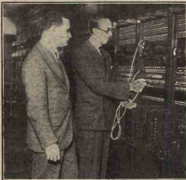
The switchboard that figures in some of the most spectacular of American Simultaneous Broadcasts. And on such occasions as the broadcasting of the King's Speech hundreds of stations are linked together by this means.
