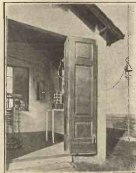
The aerial lead-in goes straight to the aerial tuner. You can see a portion of the huge tuning condenser on the left.
