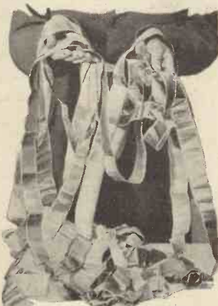
—But the "internals" of a Mansbridge type condenser, consisting of tin-foil on a paper strip.
