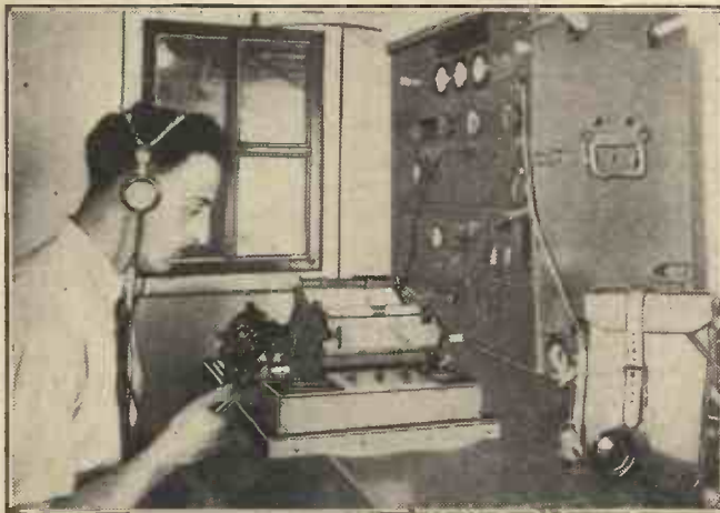
The American Army Air Corps is fitting a number of its 'planes with radio picture transmitters of the above Westinghouse pattern. They enable pilots to transmit hand-written messages and hand-drawn sketches by radio to receiving stations on the ground.
