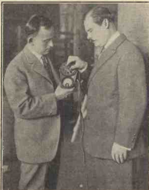
Dr. E. F. W. Alexanderson demonstrating the use of his wireless-echo altimeter.
