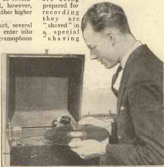
Have you tried record-radio yet? It doesn't cost much to fit up, and any old gramophone can be used, as you only require to revolve the record. Your set and its loud speaker and the "pick-up" do the rest.
