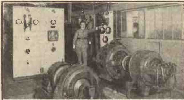
Some of the generators situated below the Eiffel Tower to supply power for the famous radio station.
