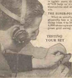
With a pair of telephone receivers connected in series with a small dry battery, you can test components for both continuity of windings and for short-circuits.
