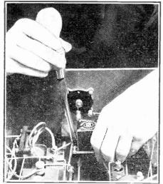
The special "Parafeed" transformer hardly takes up any space at all, and it has very useful slots on the terminal heads, enabling a screwdriver to be used for tightening up.
