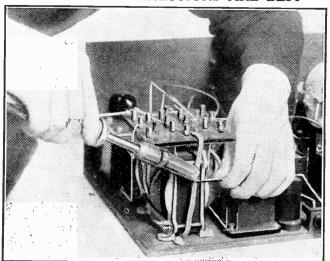
In a mains receiver it is always best to solder the more important connections, as some of them carry quite high voltages and heavy currents. If you do not feel like tackling the job, though, make sure that all connections are well screwed down.
