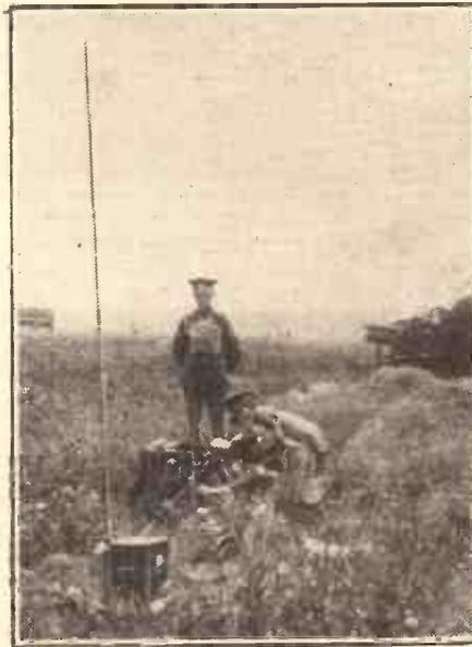
A portable field station in operation somewhere in Sussex during Army manoeuvres. Note the short, unobtrusive mast.
