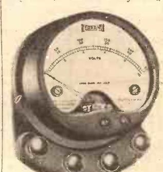
A typical triple-scale meter, the range being chosen according to the terminals used.
