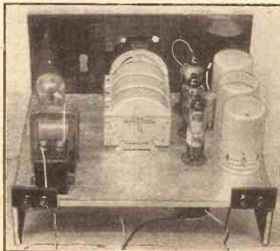
The "Double D.T." receiver seen in this reproduction was the first set with multi-mu pentodes and double-diode triode. It was designed and described by "Popular Wireless" early this year, and is typical of the clean lines of modern design.
