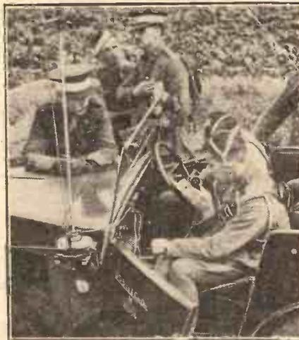
This is one of the latest mobile wireless stations manned by the Royal Corps of Signals, and used for communication between Army field units. The aerial mast can be seen on the side of the car near the windscreen.
