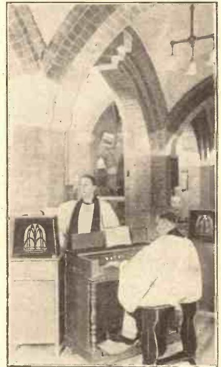
A microphone, a harmonium, a five-valve amplifier and two moving-coil speakers provide the music for St. Margaret's Parish Church, Coventry, since the regular organ broke down. The Vicar considers the tone and volume as good as that of any full-size church organ.
