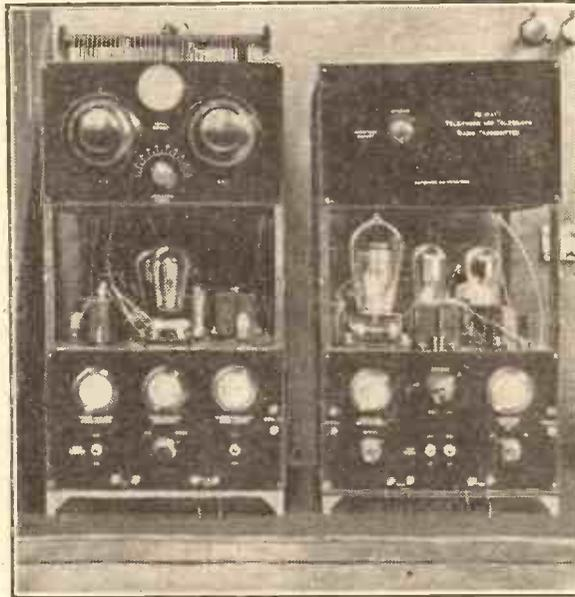
This ambitious-looking amateur transmitter is designed for C.W. or telephony operation. The unit on the left contains the crystal-controlled oscillator and power amplifier stage, while the modulating equipment is in the other unit. The transmitter is conservatively rated at 10 watts, but if necessary it is capable of handling as much as 20 watts with about 80 per cent modulation.
