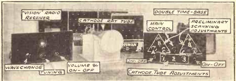
The cathode-ray system of television reception was developed by "Popular Wireless" for the home-constructor, and here you see the complete apparatus which was described in detail in "P.W." commencing with the May 27th number.
