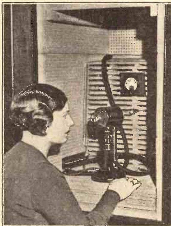
A condenser-microphone telephone transmitter at the Dolts Hill laboratories of the G.P.O. It is housed in a specially lined non-reverberating cabinet.
