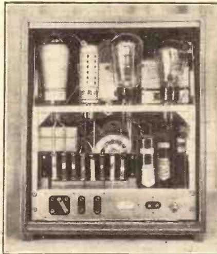
Not all commercial receivers have their small components in inaccessible places. This photograph of the new Telsens 484 receiver, for instance, shows the open and orderly arrangement of the resistances and electrolytic condensers.
