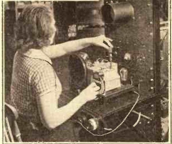
Testing a new receiver by means of a cathode-ray oscillograph in the Cossor factory at Highbury.
