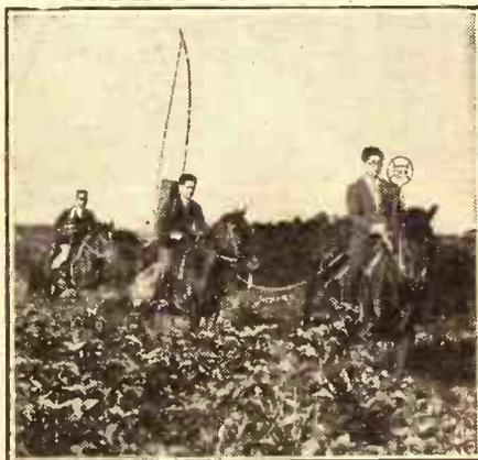
How a commentary was broadcast on Japanese army manoeuvres. The first horse carried the announcer and his microphone, the second a short-wave transmitter and the third an engineer with a check receiver.
