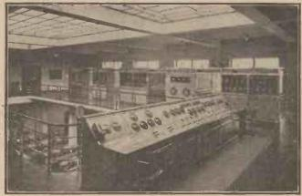
THE CONTROL DESKS allow the engineers full view of the two transmitting panels and also a good view of the generators in the hall below.
