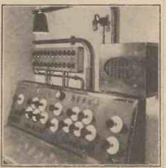
The dramatic-control panel at the "H.M.V." studios in London, with the sid of which music-and-sound effects from eleven different studios car be mixed and balanced into the making of a single record. This is the only control of its kind in the world in use for gramophone recording, and cost over £1,000. Five miles of wiring are employed in its construction.
