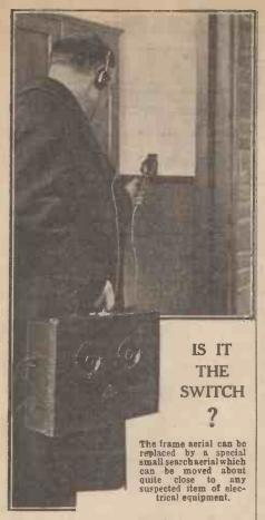
In much of the existing apparatus for locating sources of "man-made static" certain fundamental disadvantages are inherent, chiefly on account of low sensitivity and of the fact that a frame aerial built into the carrying case is used as a pick-up for the interference waves.
