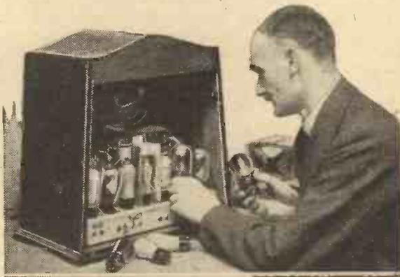
Removing the valves in a superhet so that the circuits can be tested and the valves checked over for characteristics.
