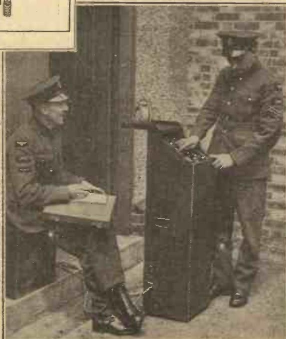
This simple-looking control-box enables the operator to make the "Queen Bee" do just what he wants it to do while it is manoeuvring in the air.
