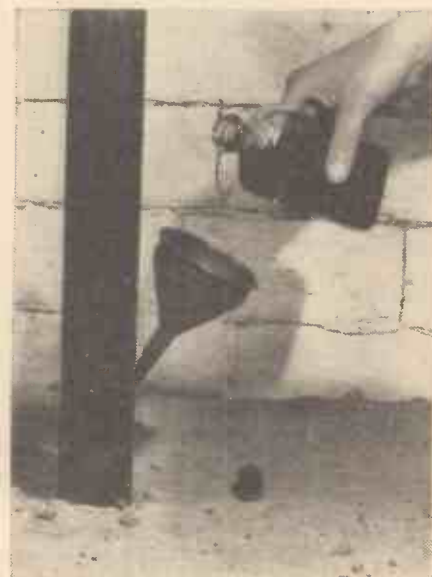
The creosote is poured into the hole in the base of the mast at intervals of a month or six weeks.
