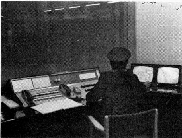
Local monitoring facilities are provided at Heathrow Central and platform-only monitoring of all three stations is provided for the line controller situated at Earls Court.
