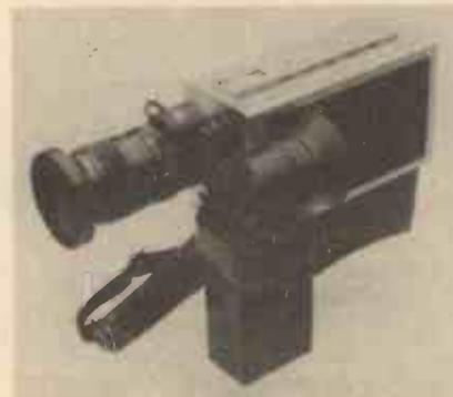
Video cameras from Ferguson can be powered from their Videostar portable cassette recorder as well as mains. The monochrome camera has a 2 to 1 zoom lens, automatic iris,
