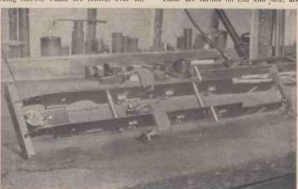
Fig. 10.—The finished main frames with buffer beams and displacement lubricator in position
