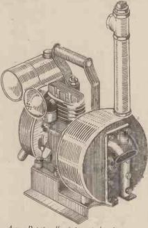
A new Batwin self-priming petrol engine pump
