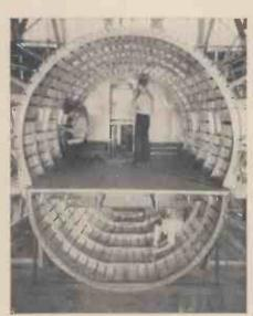
A cross section of the pressurised fusclage slowing two eccentric circles intersecting so that the floor joins their points of intersection
