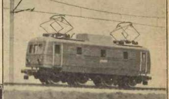
Fig. 5.- A model that has been built before the prototype. A new design for an electrically-driven locomotive for the German National Railways is demonstrated in this gauge 00 model, but the actual locomotive has not yet been built for service.
