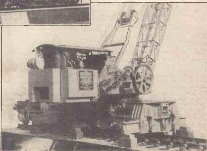
*Fig. 1.—This huge working model of a Craven Railway Service Crane is one of the most spectacular built by the late Mr. S. J. Ward. It is to a scale of 1/10th full size.*
