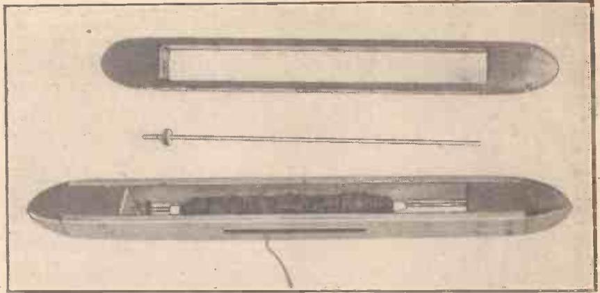
Details of a shuttle body, and a view of a finished shuttle.
