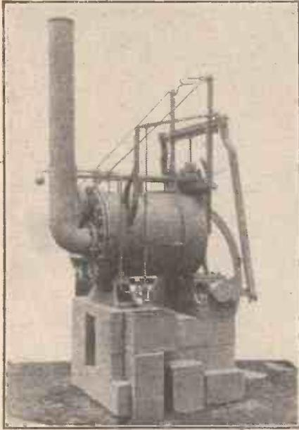
Fig. 1.—Trevithick engine and boiler. The direct-acting high pressure steam engine, patented by Trevithick in 1802 for stationary and locomotive use, eventually superseded the beam engine. This engine, found at Hereford in 1882, was made about 1805 and probably developed 7 h.p. with steam at 50lb. per sq. in.
