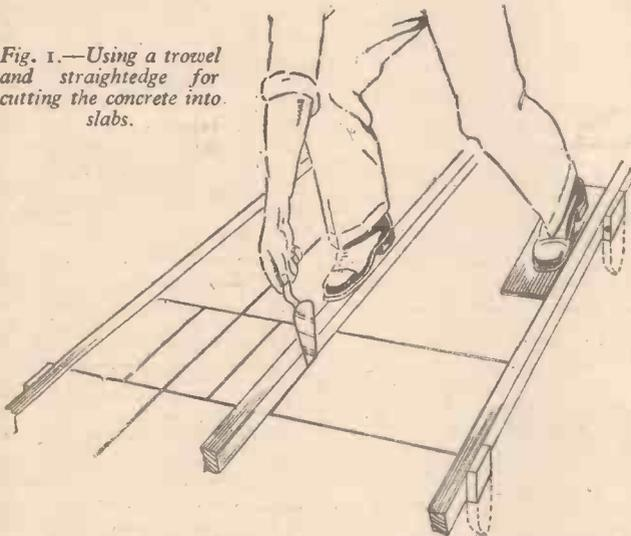
cases, as for all slab work, is three parts sand to one part cement.
