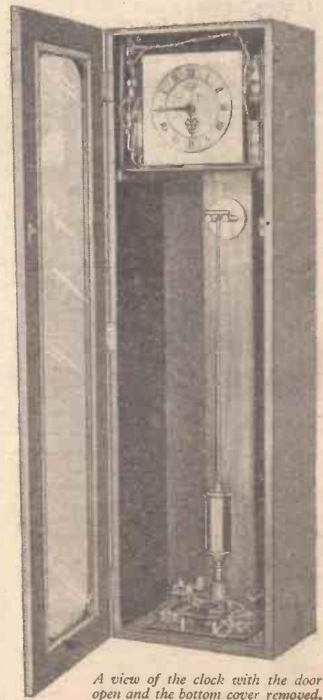
A view of the clock with the door open and the bottom cover removed.
