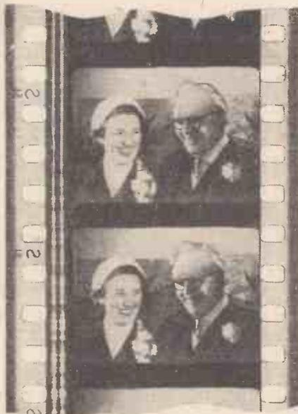
Fig. 1.—A strip of commercial 35 mm. cinema film, showing sound track at side.
