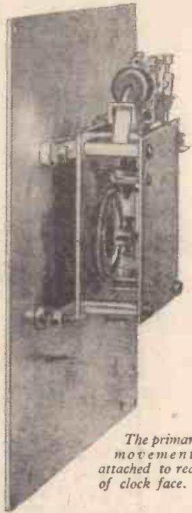
The primary movement, attached to rear of clock face.
