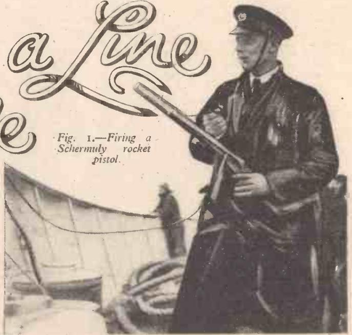
Fig. 1.—Firing a Schermuly rocket pistol.
