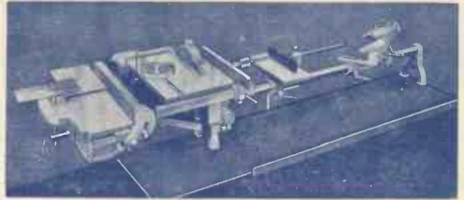
The "MINOR" lathe carrying a battery of three useful machines, any one of which may be operated without removing the others. ALL powered by ONE sturdy electric motor.
