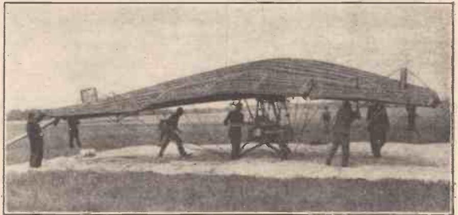
The new M.L. Light Aircraft. The novel wing construction is entirely without rigid bracing and is an inflated fabric envelope, in which pressure is maintained to provide a stiff aerodynamic surface. The plane, with wing collapsed, is towable behind a private car.
