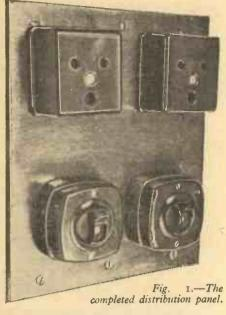
MATEURS who use the kitchen as a darkroom will, usually, have only one electric outlet available. Normally this is used for a vacuum cleaner, a small fan, or a radiator. In some cases the socket of the kitchen lamp provides the one and only outlet, and using this can be dangerous as no earth connection is provided as with
