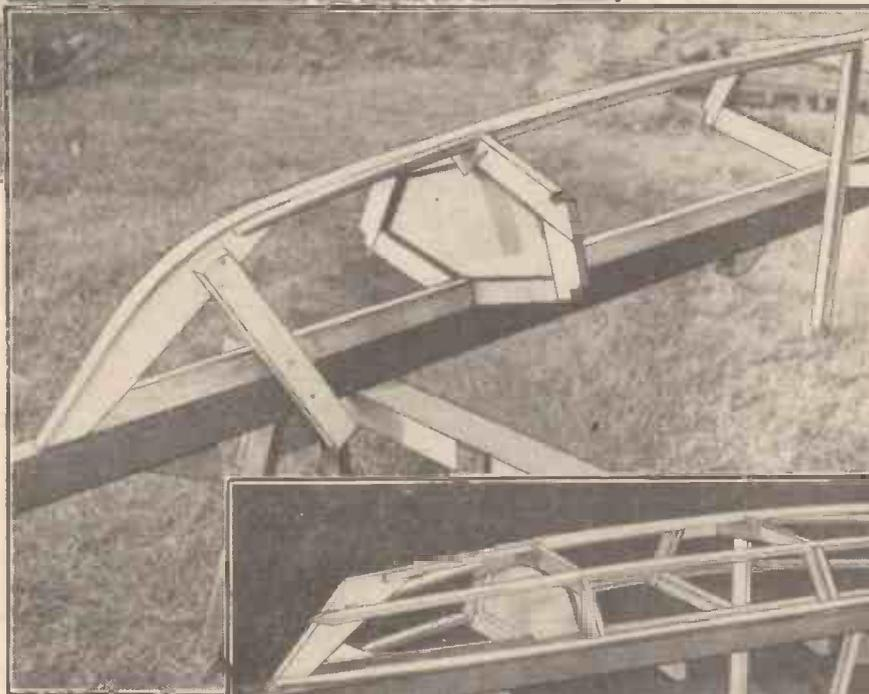
Fig. 13 (Right).—A chamfer is worked on the bow and stern post before adding the chine and sheer strips.
