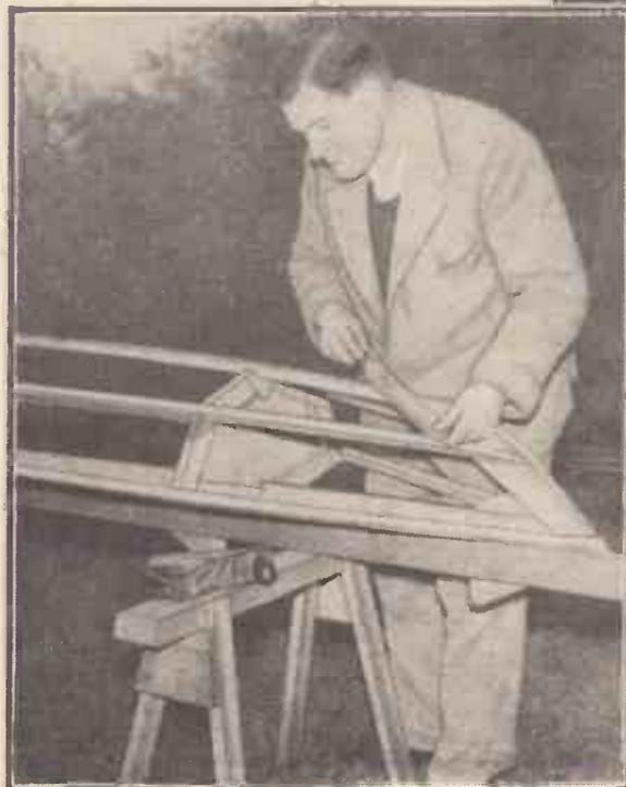
the correct position, start nailing with some 3/4in. flat-headed brass escutcheon pins. Space the nails about 2in. at first and then fill in later at 1in. intervals. At the points of greatest strain it is helpful to use one or two 3/4in. X No. 2 brass countersunk head screws as these will not draw out slightly which might well happen with the nails alone.
