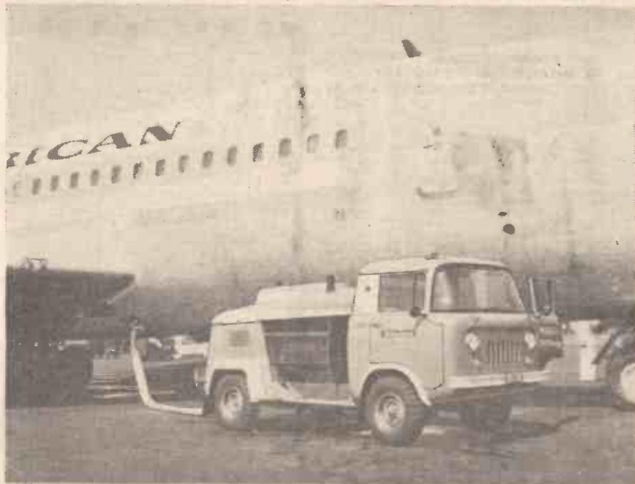
Designed for starting jet engines, air conditioning aircraft interiors and de-icing operations, this surge-free rotary screw compressor known as the Atlas Copco Air Partner will help to ensure on-time departures of aircraft. The compressor, which has no wearing parts and will run for 10,000 hours without an overhaul, is shown above starting a Boeing 707 jet airliner.
