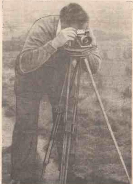
Fig. 5.—Set up the tripod with the legs well spaced.
