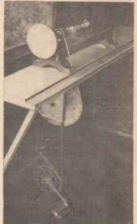
Fig. 2.—The completed pedal powered lathe.
