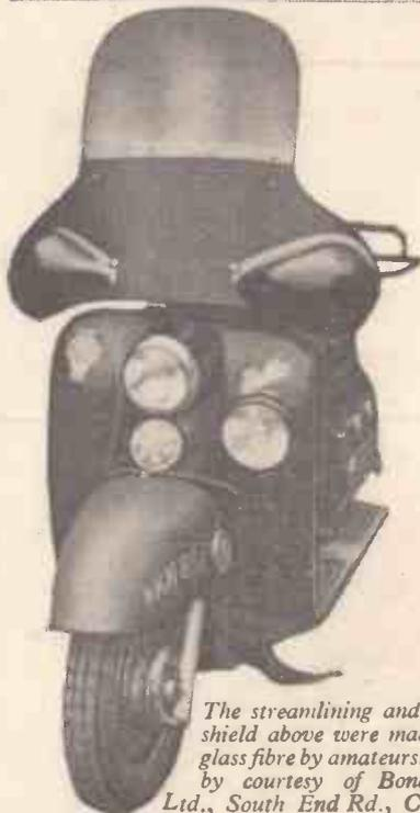
The streamlining and scooter shield above were made from glass fibre by amateurs. Photos by courtesy of Bondglass, Ltd., South End Rd., Croydon.
