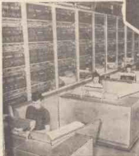
Fig. 1 (Above).—The automatic letter sorting machine being used in a Washington post office.
