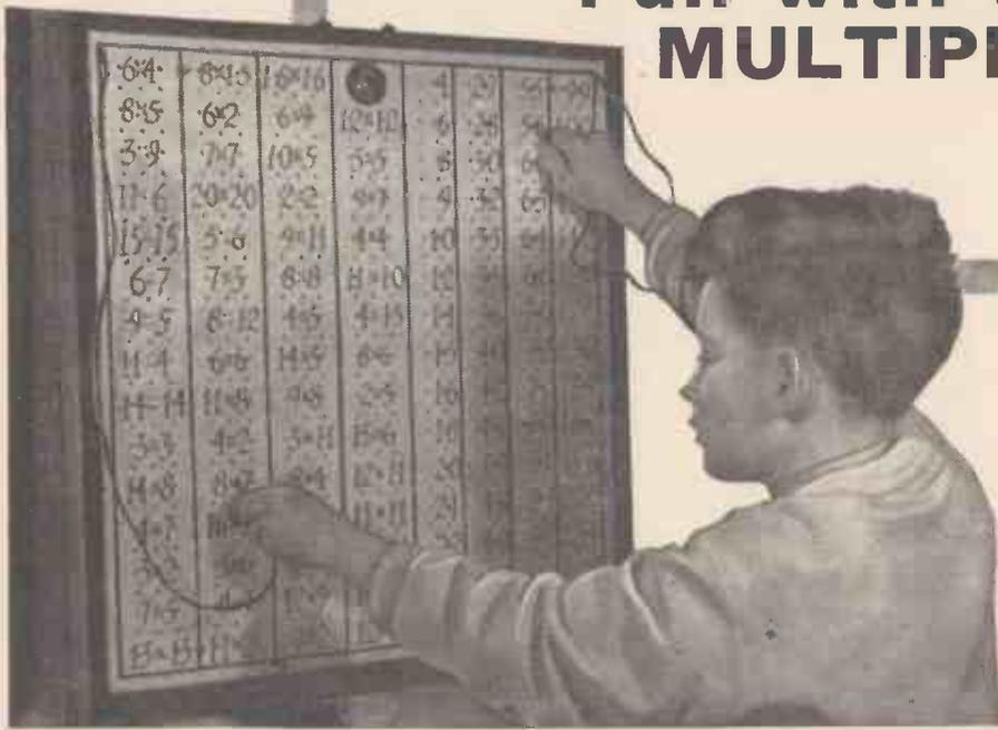
THE construction of the board is a simple matter and is based on the idea of a bulb being lit up when a correct answer is given. By using interchangeable boards, there is no limit to the variety of
