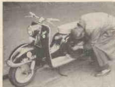
Fig. 2.—Checking the air cleaner.
