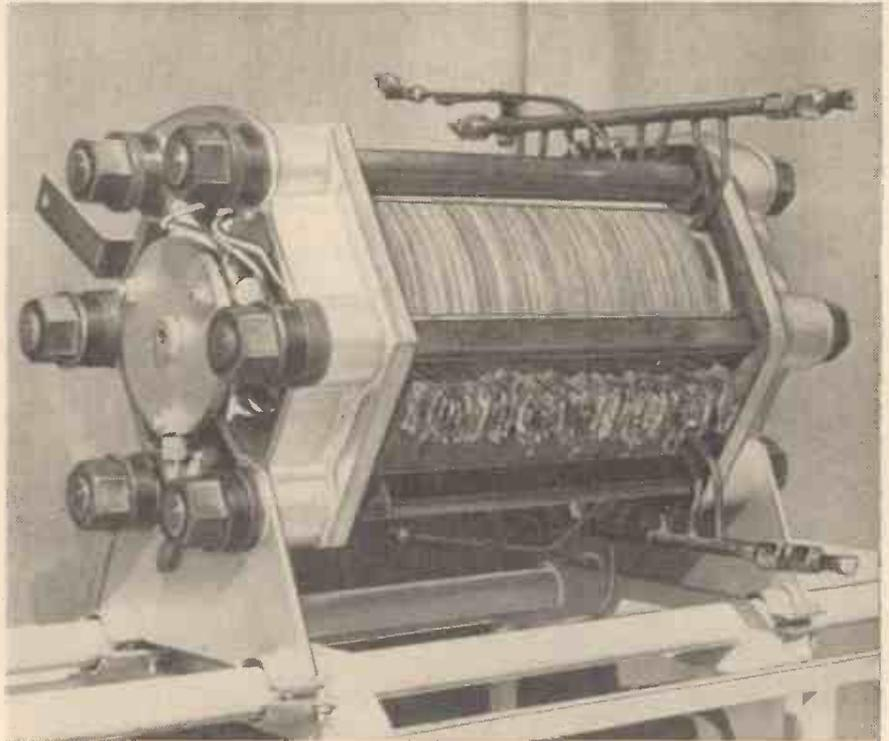
A 3kW. power unit utilising 40 hydrogen/oxygen cells linked in series.
