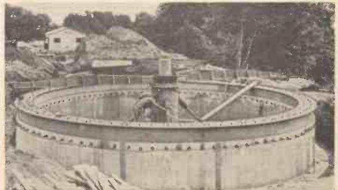
Fig. 3.—The base for a low-noise horn antenna under construction at the satellite communication station site at Holmdel, N.J.
