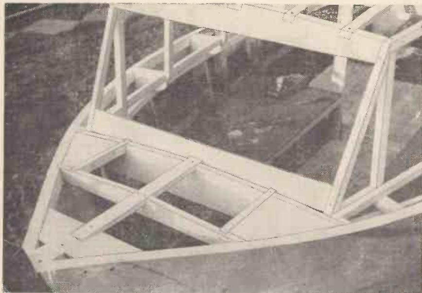
Fig. 23.—The fore deck framing.
