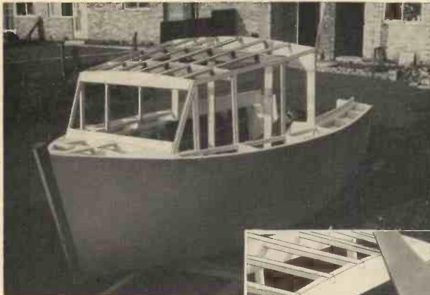
Fig. 30.—A photograph taken during cabin construction.
