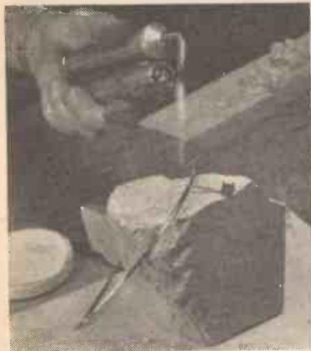
*Silver soldering in progress. The headband is supported on a piece of refractory brick. The joint must be well coated with flux before heating.*
