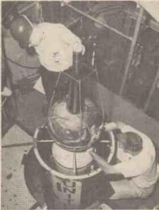
The Vanguard satellite is installed atop the satellite launching Vehicle 7 at Cape Canaveral.
