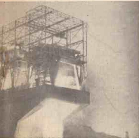
The cooled portion of the thrust chamber is 11ft. long, 40in. in diameter at the throat chamber and 9½ft. in diameter at the exit.
