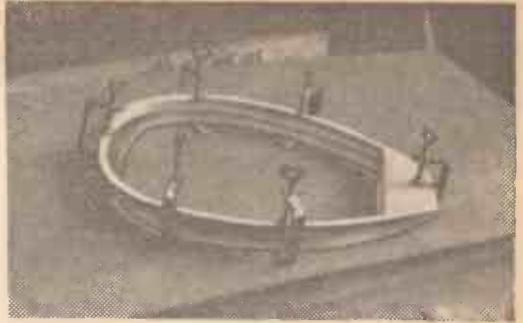
Laminations are clamped and glued together in pairs.
