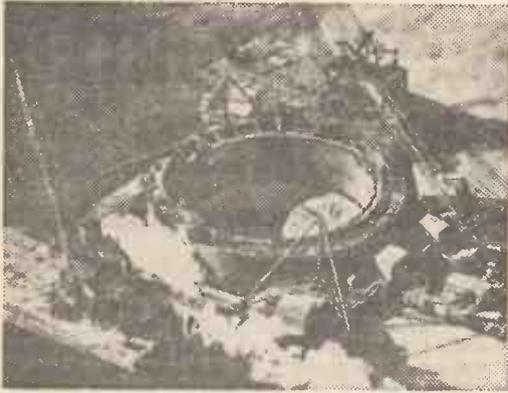
This is a circular steel caisson sinking down into the mud beneath the waters of the Straits of Mackinac in the United States. Barge mounted cranes dig out the mud from inside the caisson whilst the sides are slowly built up.
