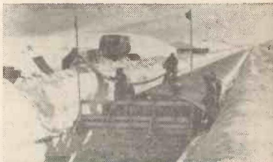
*The second step . . . Installing archways in the excavated trenches.*
