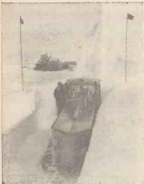
*The first step in the preparation of a city under the ice. A snowmill cutting one of the many trenches of New Byrd.*
