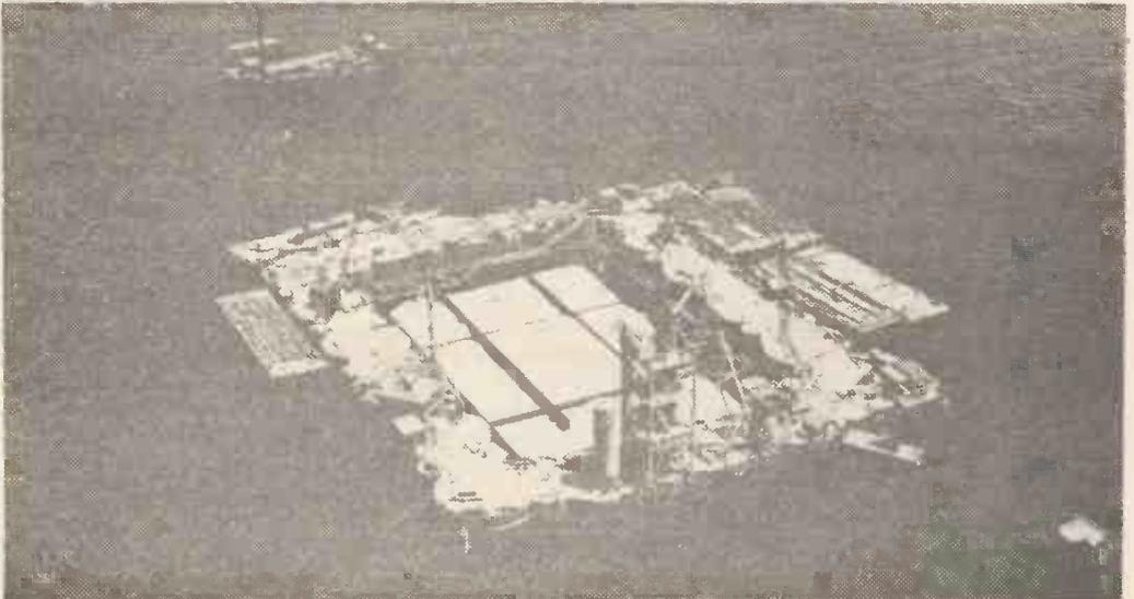
A temporary wall has been built around the site of this bridge foundation, the water pumped out and the cutting edge of the rectangular box caisson assembled on the dry floor. Slowly it will sink down through the mud, the sides being added to all the time, to keep them above the surface.
