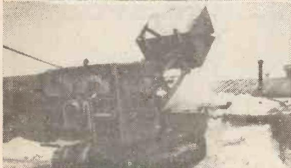
*D-4 Traxcavator filling the snow melter at McMurdo Sound base.*
