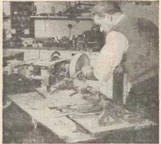
Fig. 8.—Providing chisels are kept sharpened the inside can be worked fairly rapidly, move the tool-rest closer as cutting proceeds.
